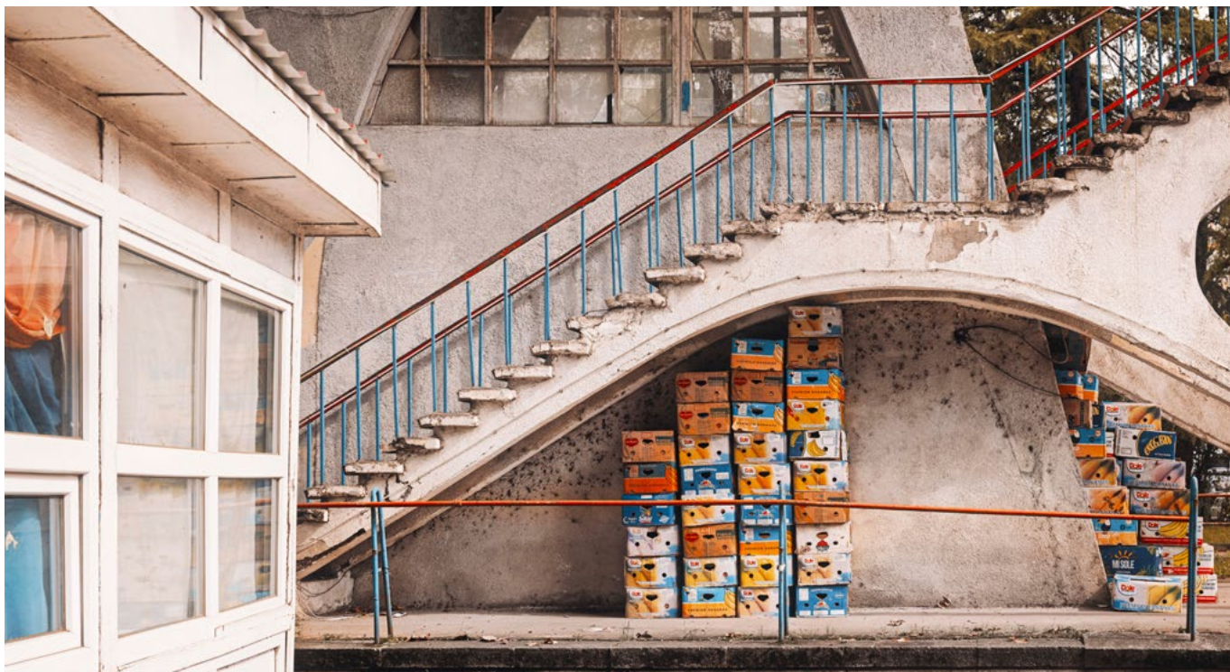
Another part of the Chiatura cable car infrastructure.
